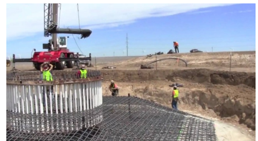
PáTu Wind Farm construction
