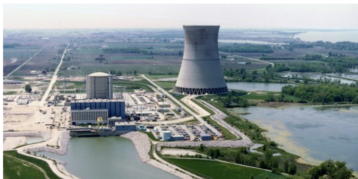
Davis-Besse nuclear plant
